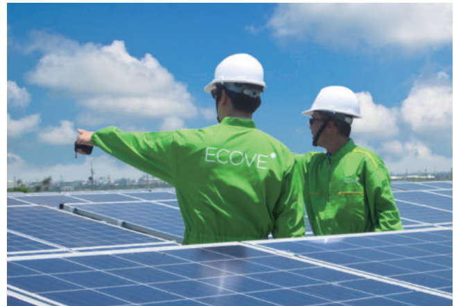
▲Image 27 / Installing a photovoltaic system
